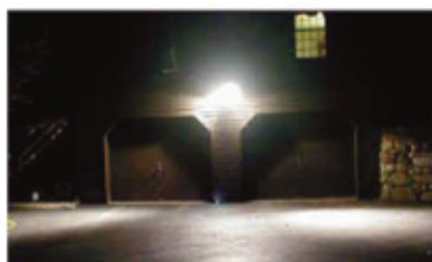
Poor Lighting—directed upward
