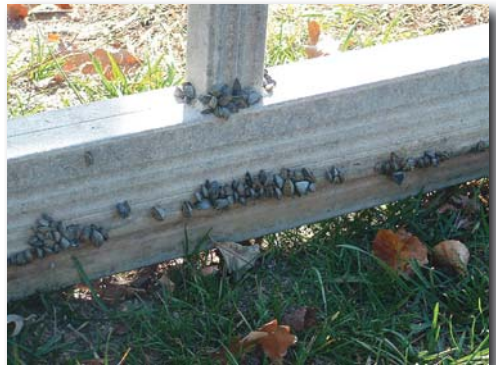
Zebra mussels attached to lift
