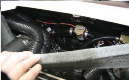
Ballast system water pump, water lines, and caps should all be flushed and cleaned.
